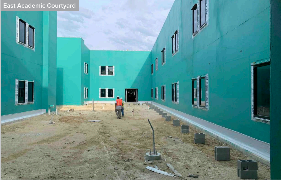
Aluminum Storefront Installed
